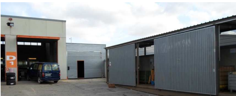
Box Services (Workshop D1) and Waste Collection Point
